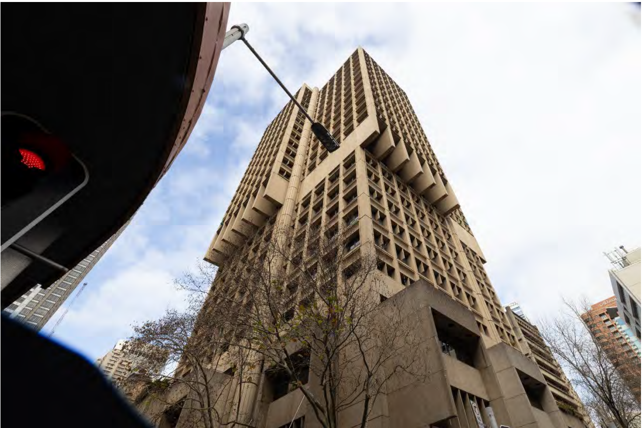
Image 3. Exterior of Town Hall House. Photo by Abril Felman / City of Sydney
